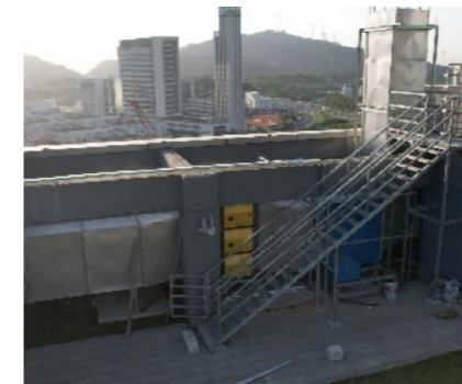
Cooking Fume Discharge Outlet After Rectification
