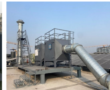
Waste Gas Equipment Reconstruction
